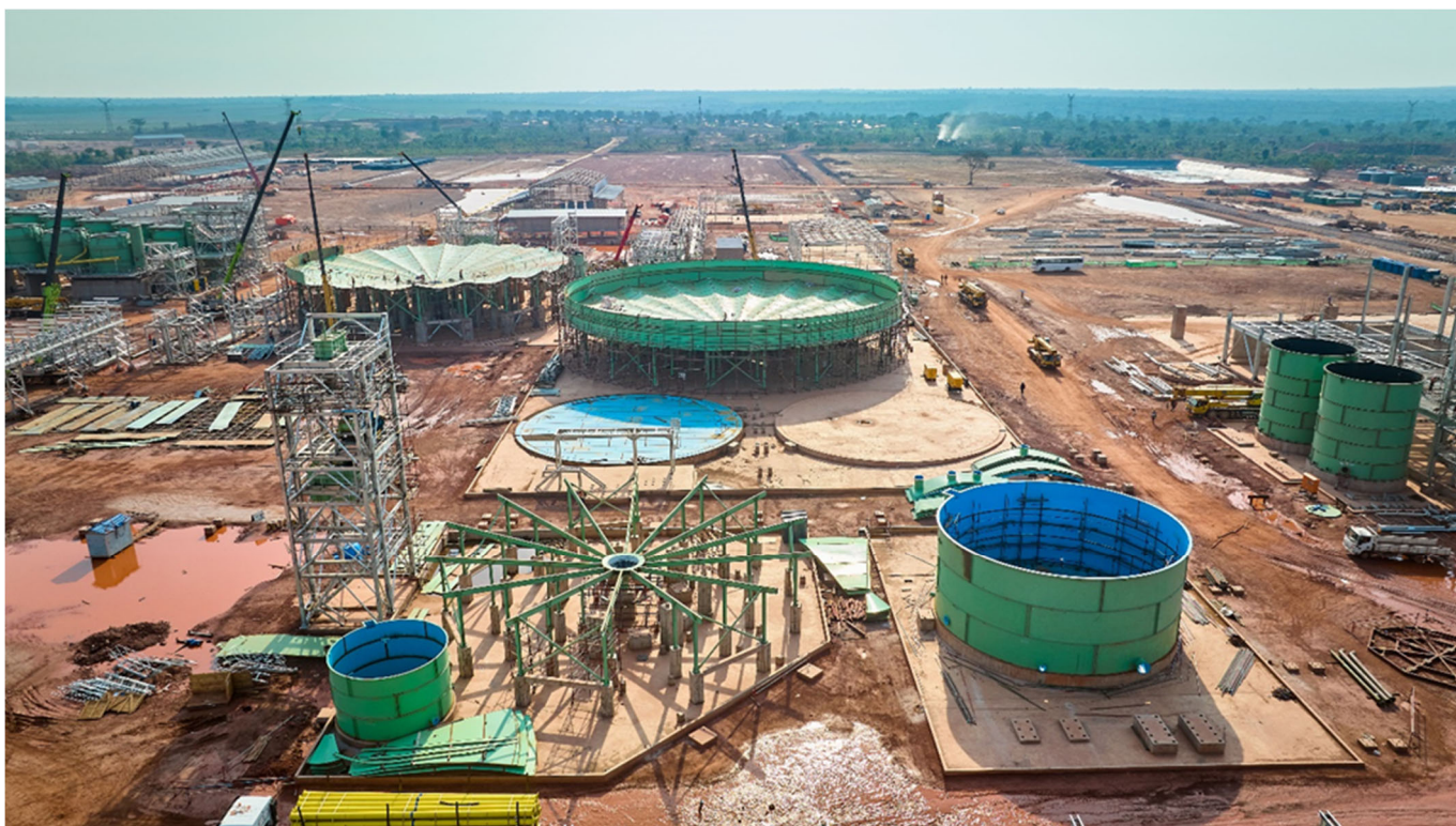
Photo: Construction of the concentrate thickener is progressing well at Kamoakakula's Phase 3 concentrator site. The process design of the Phase 3 concentrator is very similar to that of the Phase 1 and 2 concentrators, but 30% larger.
