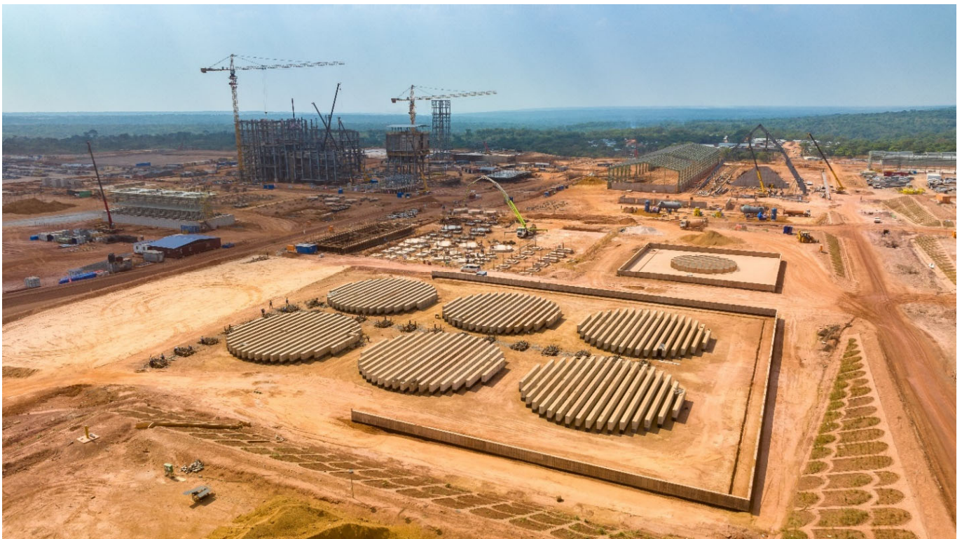
Photo: The foundations and civil construction for the Phase 3 smelter's high-strength sulphuric acid storage tanks are now complete. As a by-product, the smelter will produce between 650,000 to 800,000 tonnes per year of high-strength sulphuric acid, which is planned to be sold domestically.
